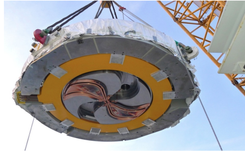
Installation of the Proteus-235 cyclotron at IFJ PAN
